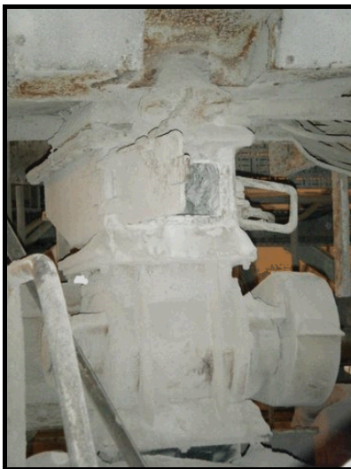
Inspection hatch shown in the open position
