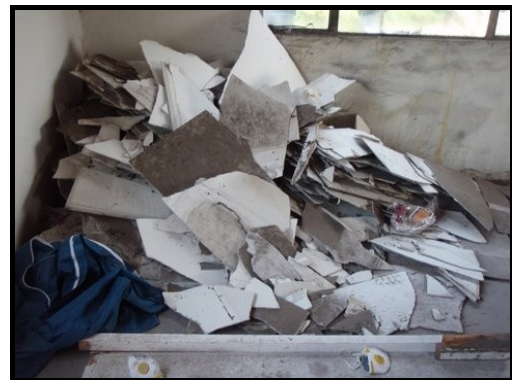
Pile of asbestos debris left in a corner of the building
