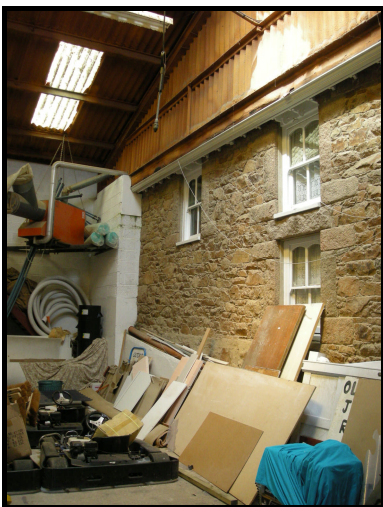
Area into which the person fell
